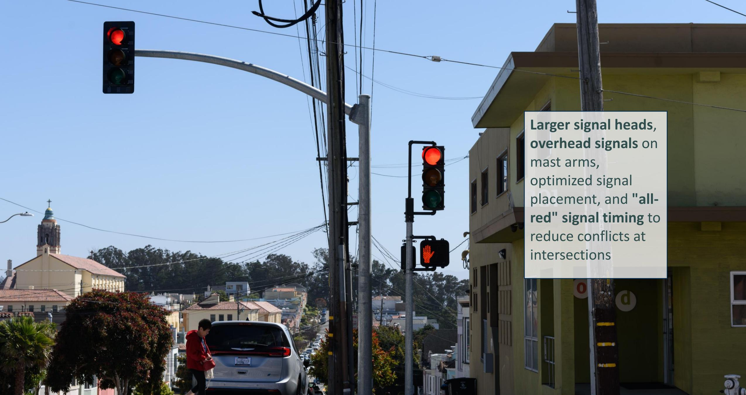
Larger signal heads, overhead signals on mast arms, optimized signal placement, and "all-red" signal timing to reduce conflicts at intersections
